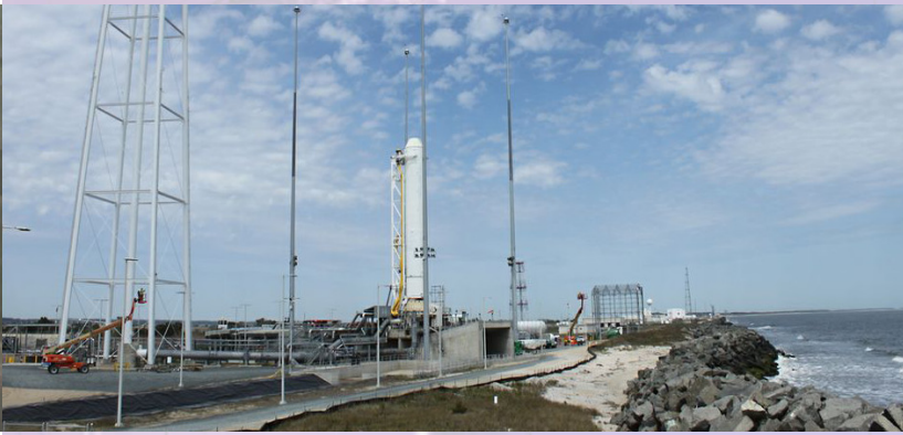
December 2012: Antares launch pad completed at Mid-Atlantic Regional Spaceport.
